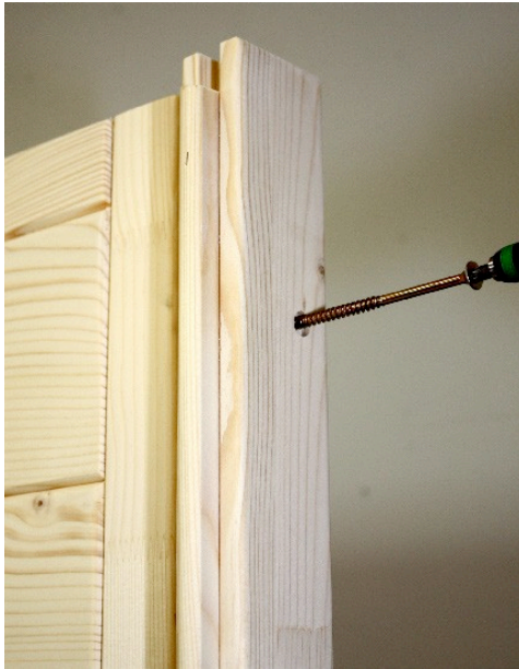
8 screws 6 x 120 mm per corner post
